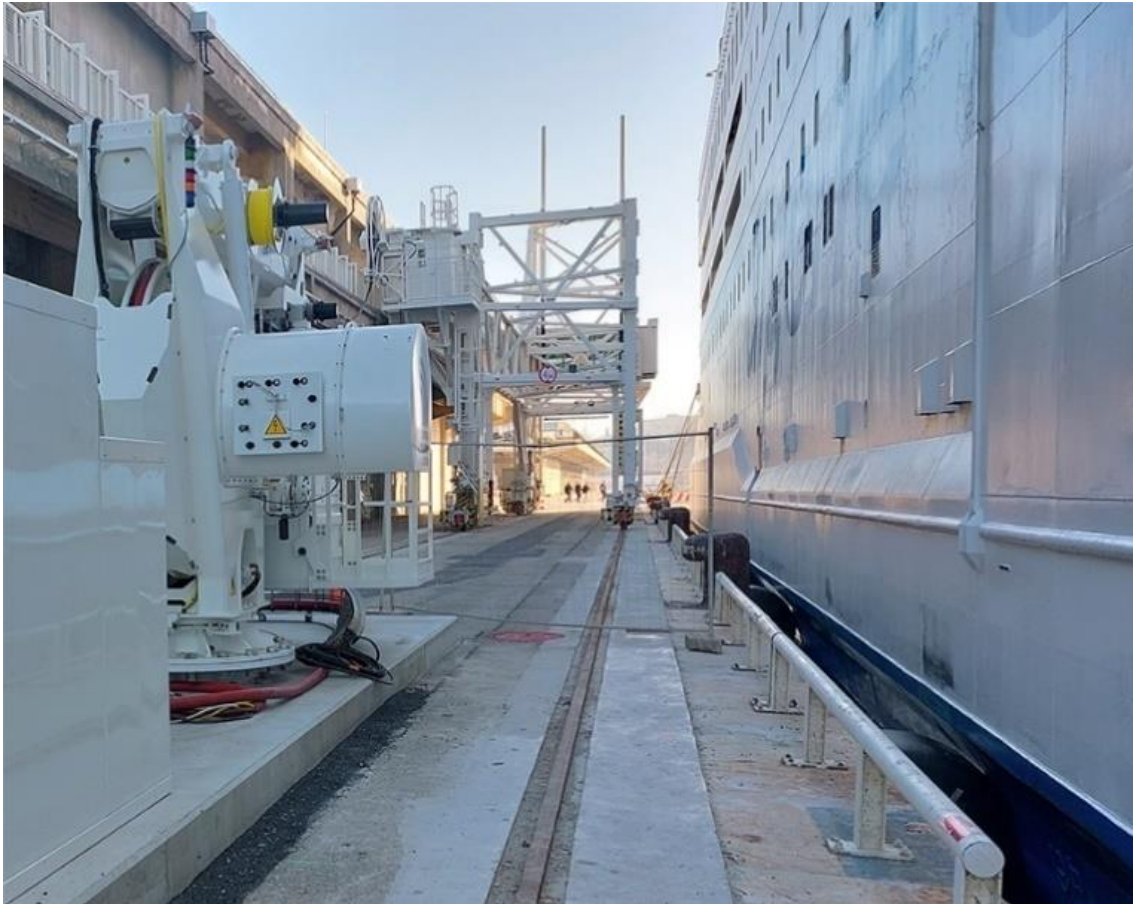
Figure 72: Shore power connection - Marseille
